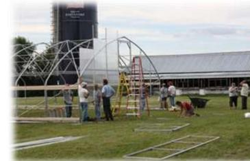
End walls hung from end bow by sections. Vent section first, two sides next. Doors can be hung after polyethylene is on structure.
