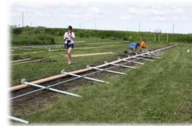
Track inspected to be sure there are no low spots. Ground anchors placed on outside of tunnel for entire length (both tunnel positions).
