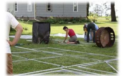
Stand up side walls to prepare for installation of bows. Ladders in the center at each bow help stand bow up and into receiving poles of side walls. Side wall cross braces used to hold sides up.
