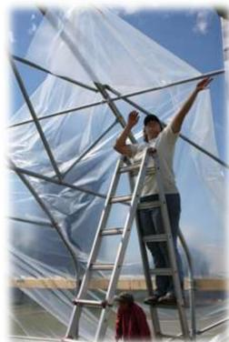
Inside the tunnel, preventing hangups as poly is pulled over. Two people on ladders was adequate.
