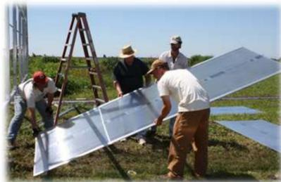
Standing up an end wall section. Attached to outside bow. Multiple people to hold wall in place is useful.
