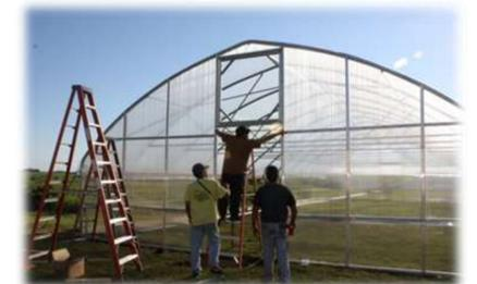
Hinged entry doors (removable pin hinges recommended), tilt up doors at bottom of end wall and vents put on last. Step up drill bit handy for piloting holes in metal useful.
