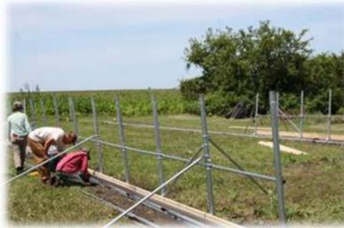
Bows are put together on ground. Lifted over one side wall and slid into receiving poles on side walls. Start on one end of tunnel and work towards other end, installing purlins as each bow goes up.
