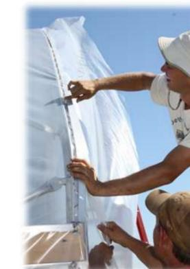
Wiggle wire inserted into channel to hold plastic in place. Excess plastic is trimmed. One end attached first, then pulled tight before 2nd is attached.
