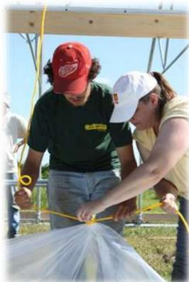
Tennis balls and rope to pull 6-mil polyethylene plastic over the high tunnel.
